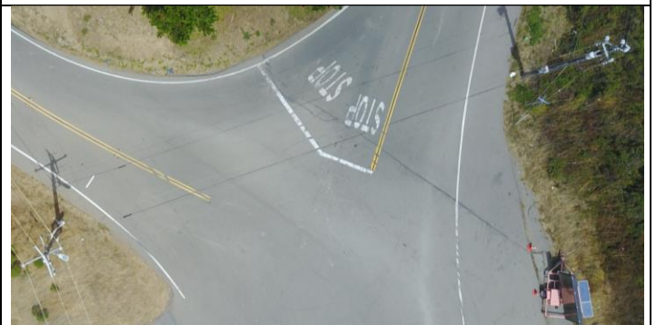
Sequoia Valley Road approach is (unnecessarily) very wide with two STOP pavement markings. Panoramic Highway SB approach is not aligned with Panoramic Highway to the south, but points directly to east to road shoulder, rather than bending naturally towards the south.
